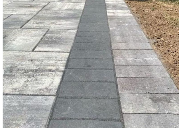
Pavers and paving band
